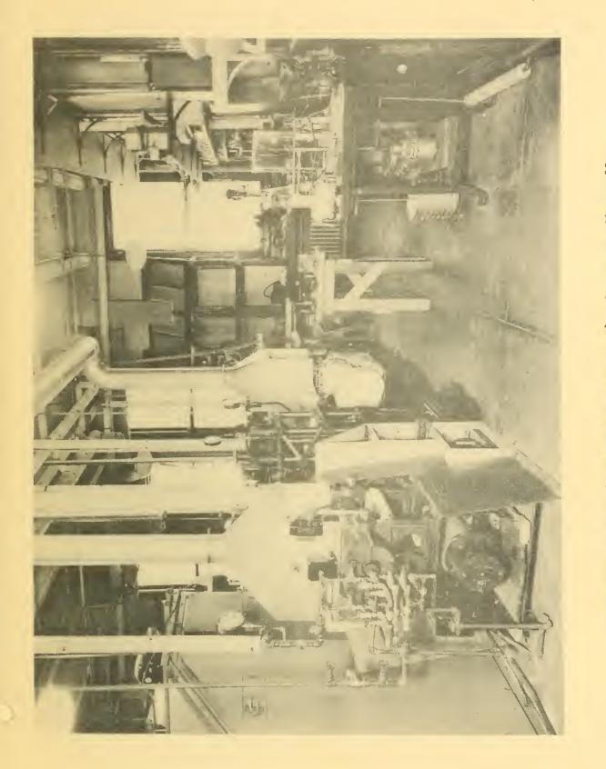
Beginning at left (clockwise around room): 1. Compounding rolls. 2. Hydraulie press. 5. Mixer. 4. Plastics flow tester.
